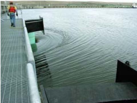
Water flowing at the top of the wier.
