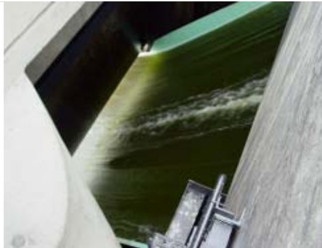
Looking down the wier from the side.
