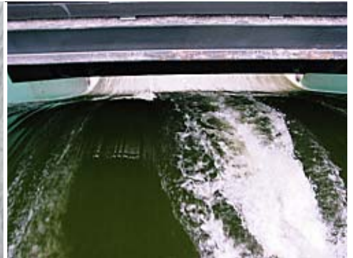
Looking directly down the wier.
